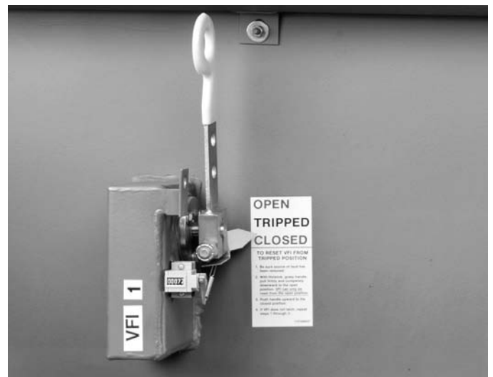
Figure 4. VFI operating handle, three-phase ganged operation. 931158KMA
